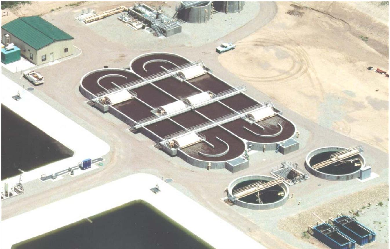
**Figure 3 ~ Oxidation Ditches with Lakeside Aerators**
